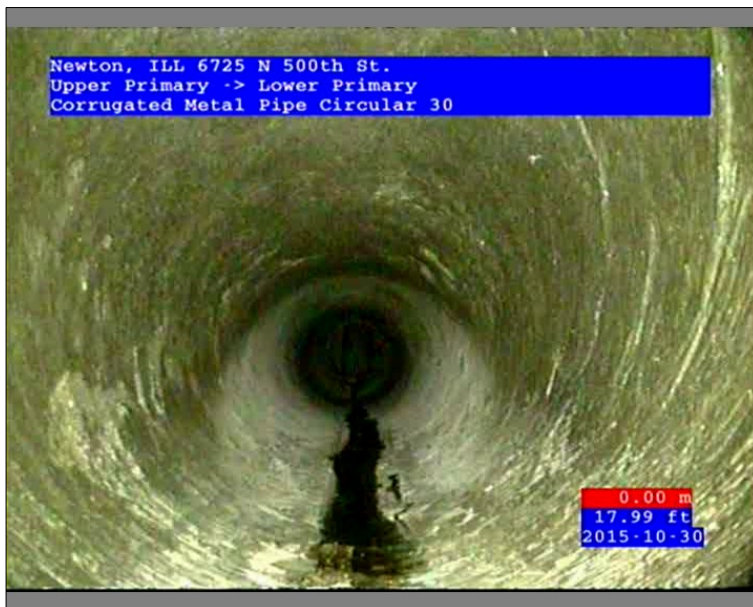
Photo: 45602-103015-01-AECOM Denver-1-30102015110025_A.JPG 17.99FT, General Observation / Reached Clients Needed Footage
