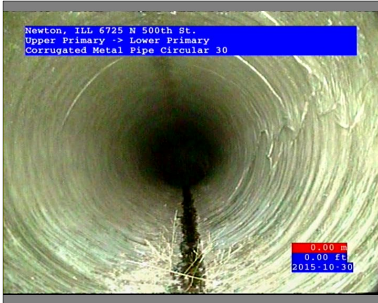
Photo: 45602-103015-01-AECOM Denver-1-30102015105328_A.JPG 0FT, Special Chamber / Survey Begins @ Upper Primary
